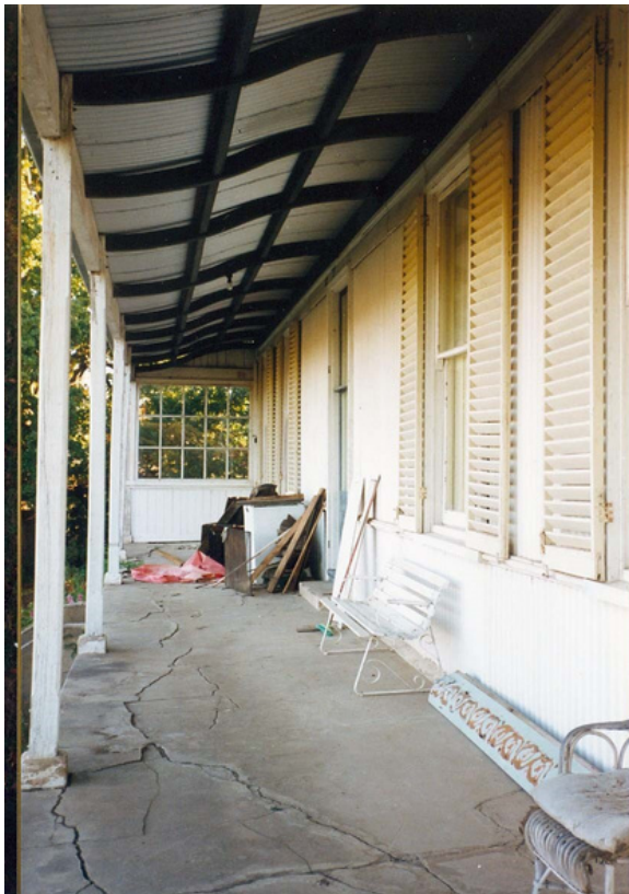
Wingecarribee, verandah view: Miles Lewis.
