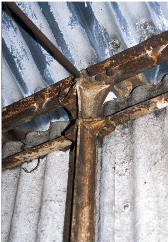
The Fitzroy Depot building before removal, head and foot of a stanchion: Miles Lewis.
