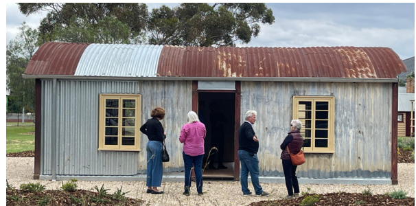
PBWHNTF visits iron on building, Keilor #087, 1st February 2022 Natica Schemeder (City of Brimbank heritage adviser), Janet Beeston, Arthur Andronas (heritage architect), Mary Lewis: Tony Isaacson
