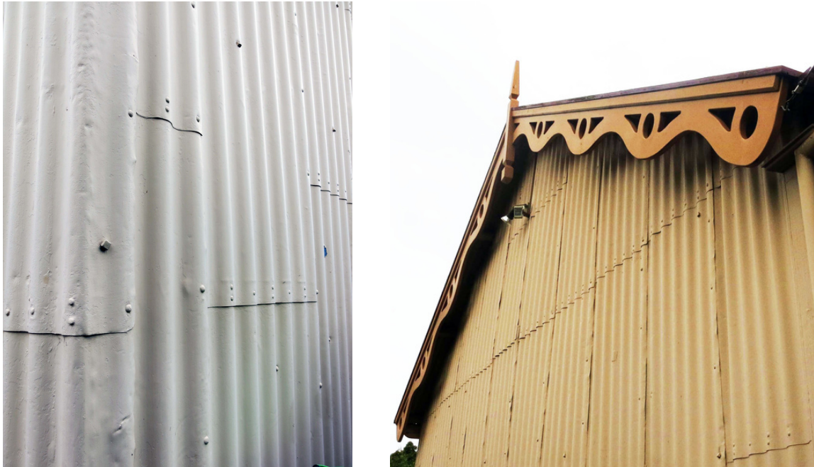
189 Brunswick Road, north wall cladding and gable: Miles Lewis.
