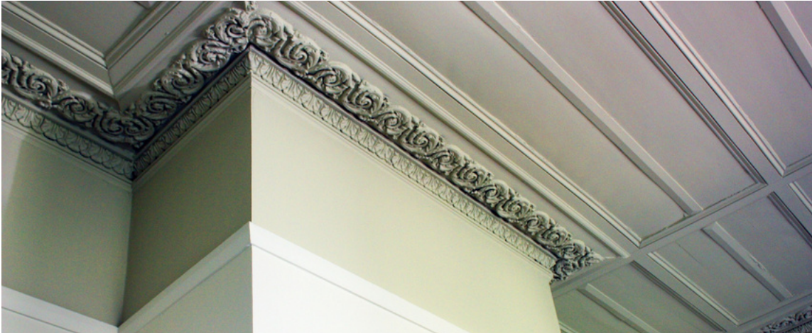
Wingecarribee, a panelled ceiling with papier mâché border and cornice mould: Miles Lewis.
