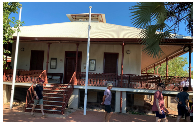
Broome Cable Station, now Court House, 2022: David Hogg
