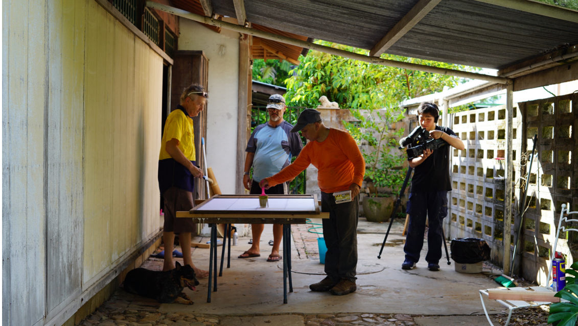
Master builder Akira Mitsuda restoring shoji screens on site: Jan Cattoni.
