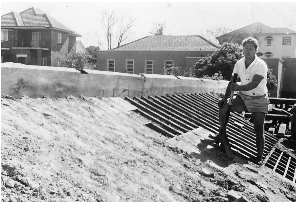
Dismantling of the verandah roof at the Brisbane site in 1962, showing the construction of round pole rafters, transverse boards, and mud, onto which the tiles were laid: Markwell collection.
