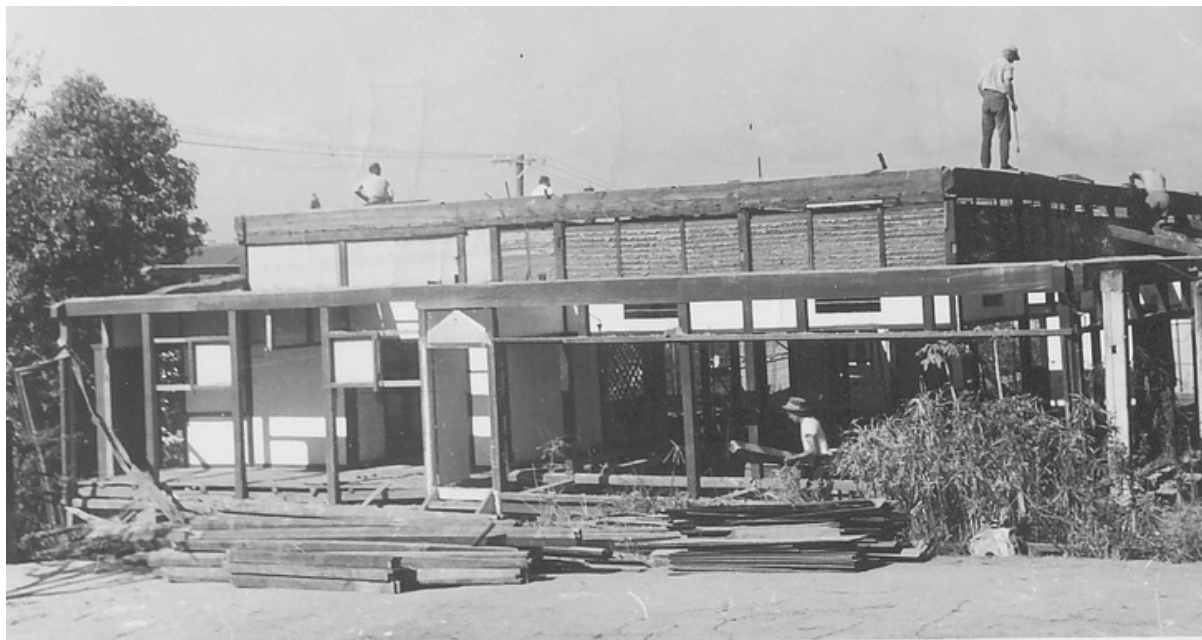
Views of the house during dismantling: Markwell collection.
