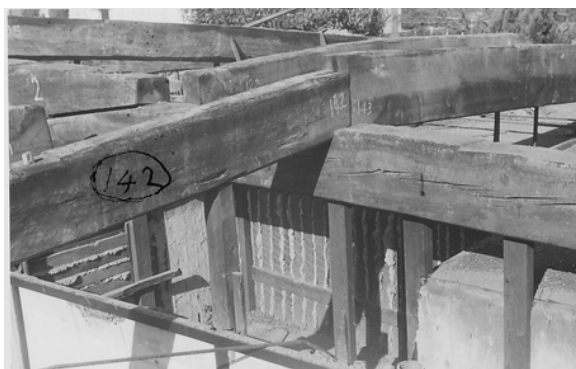
Views of the house during dismantling: Markwell collection.
