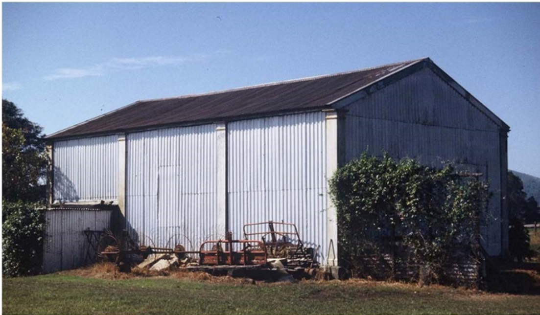
Iron church at Numbaa: Miles Lewis
