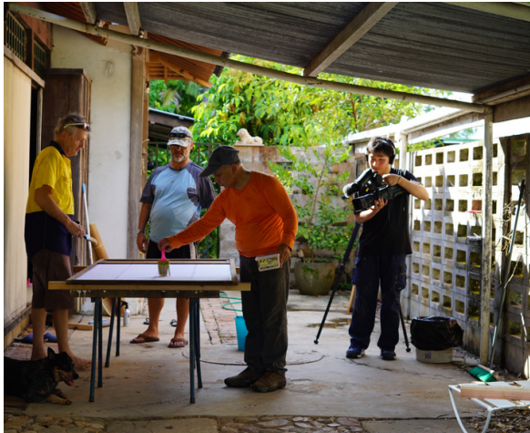
Master builder Akira Mitsuda restoring shoji screens on site: Jan Cattoni.
