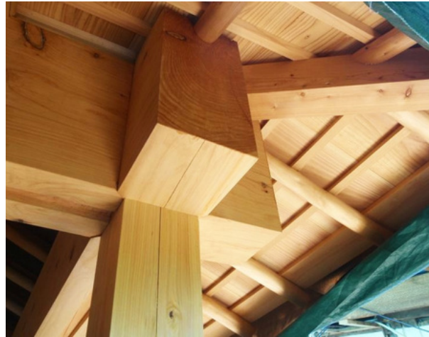
Details of restoration of the eaves and the gablet: Hugh Markwell.
