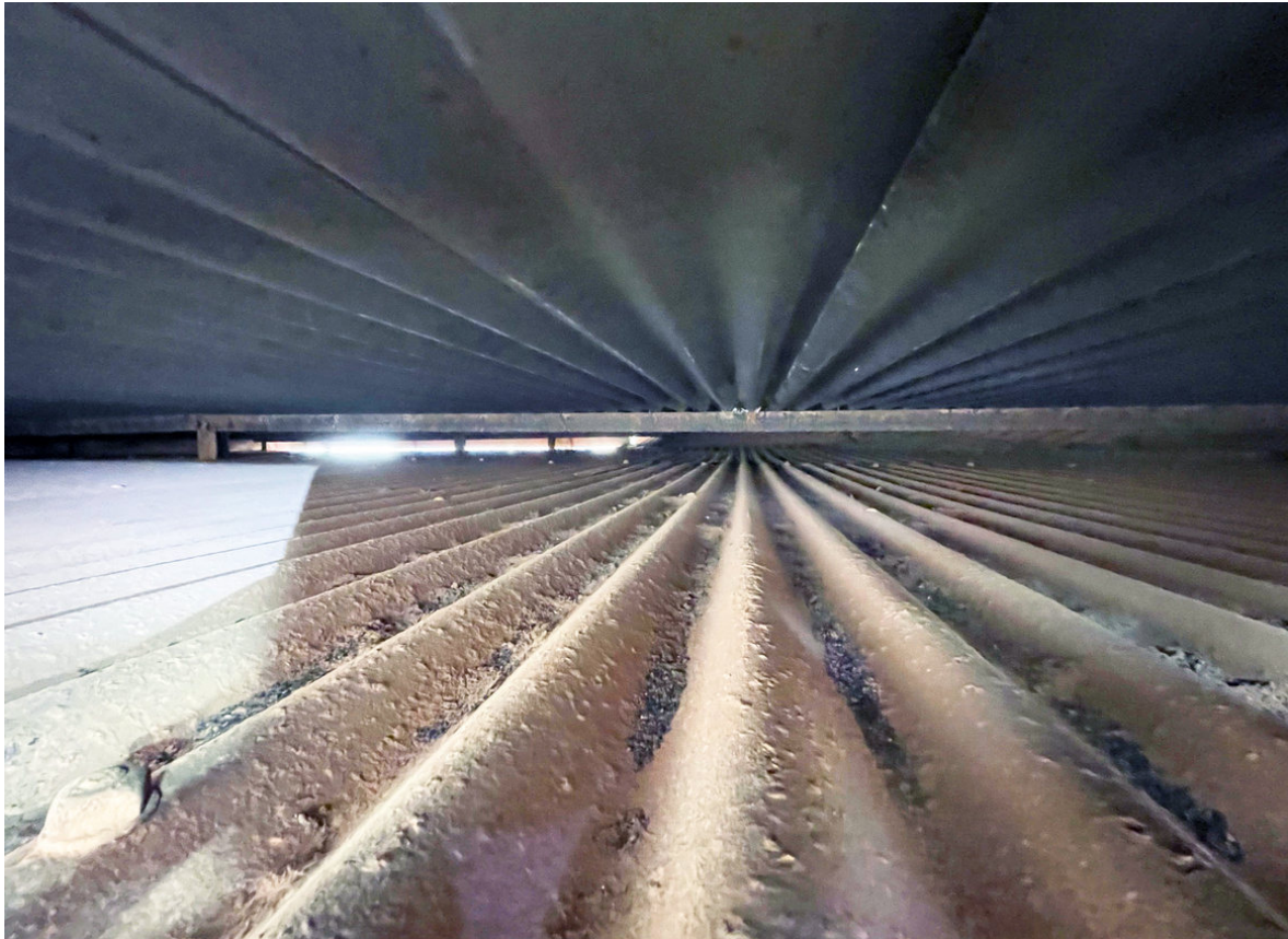
Interstitial roof space: Tony Isaacson.
