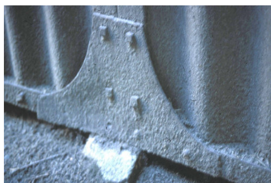
The ranger's house, Parkville, detail of the Walmsley plaque and a gusset connection: Miles Lewis.
