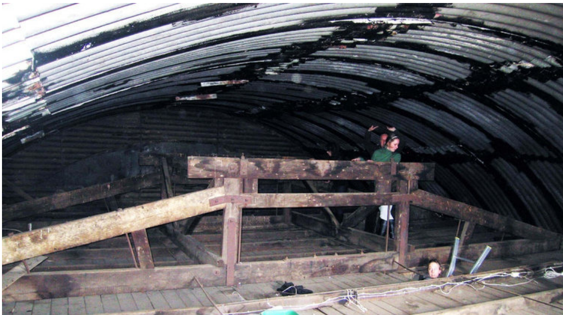
Brown Brothers store, roof space showing the queen post truss suspension system: Miles Lewis.
