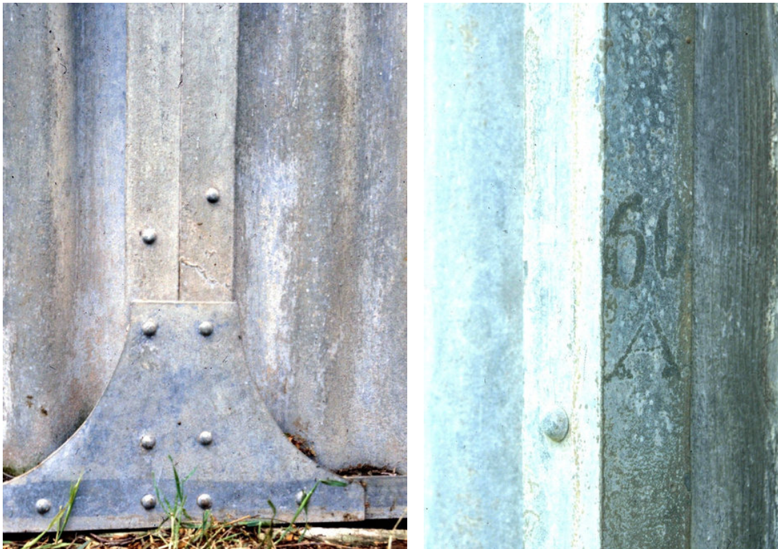
Details of the house at Inverleigh, gusset base joint, corner angle labelled '60/A': Miles Lewis.
