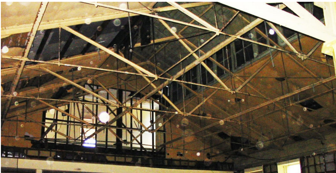
The Royal Mint, roof trussing: Miles Lewis.
