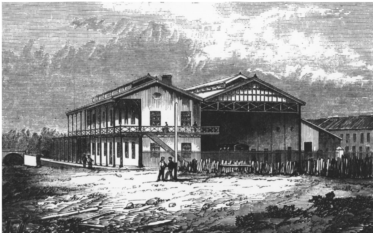
Terminal Station, Ipswich, Queensland, designed by Sir Charles Fox & Son, commissioned by J & R Fisher of Westminster, and possibly fabricated by Frederick Braby & Co, 1868. Illustrated London News , 10 October 1868, p 364.
