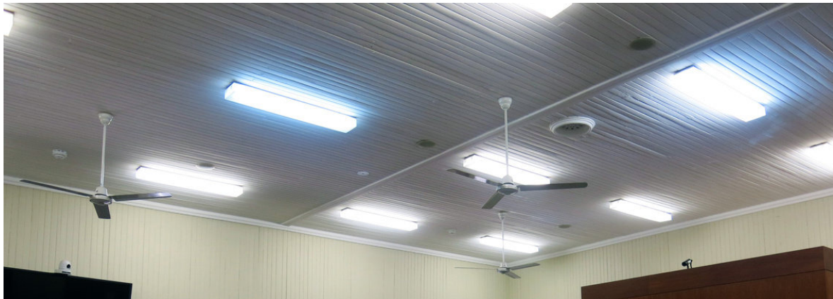
The court room, showing the cover strap which divides the ceiling in a north-south direction, not on the line of any known partition: Miles Lewis.
