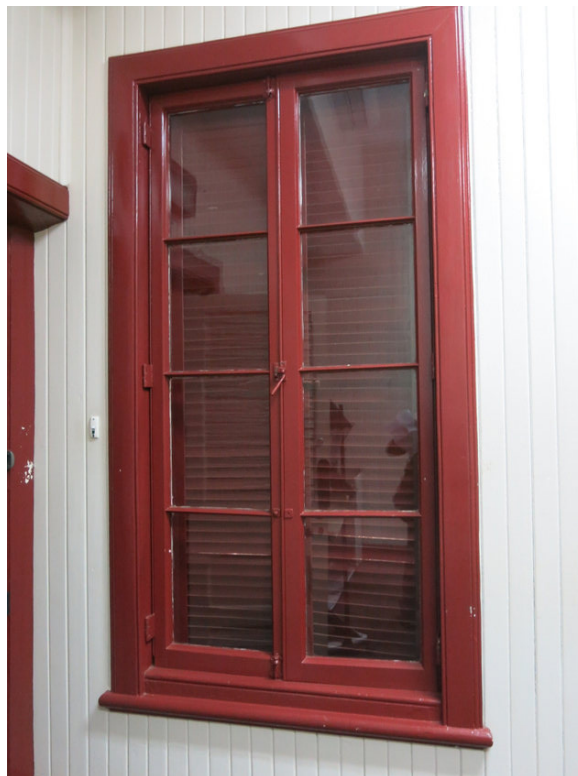
A window, interior face: Miles Lewis.
