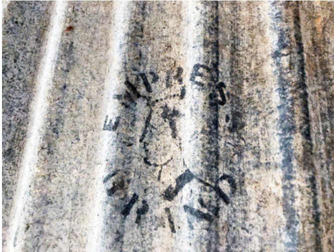
Empress brand on the lower layer of corrugated iron: Janet Beeston.
