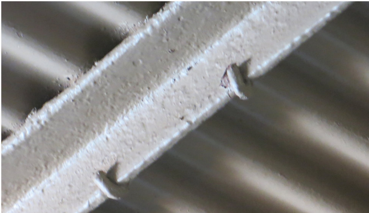
Hook bolt roof fixing: Miles Lewis.
