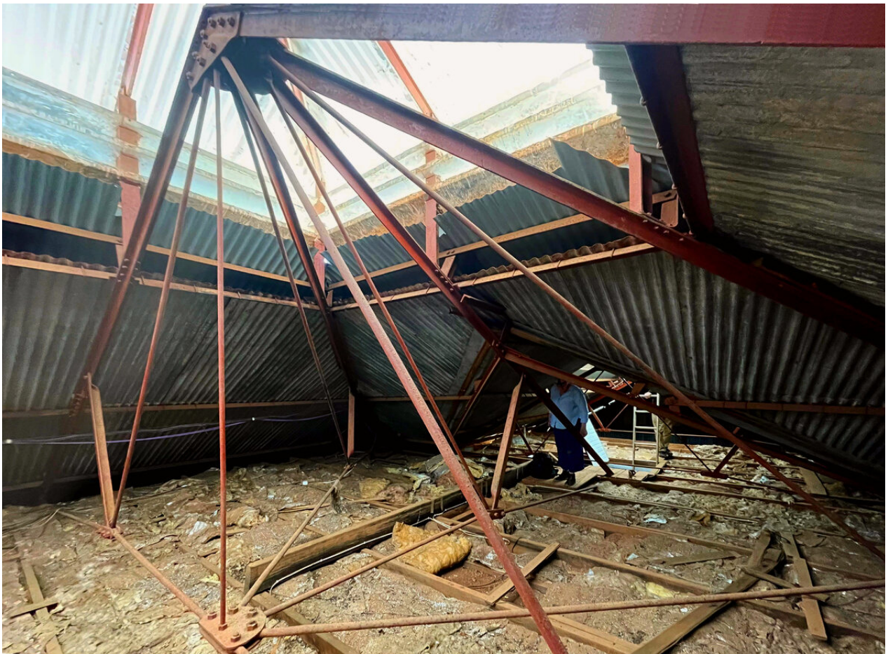
Broome Cable Station, now Court House, roof space, November 2022: Tony Isaacson.
