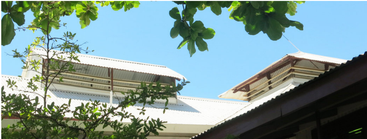
The ventilating lanterns: Miles Lewis.
