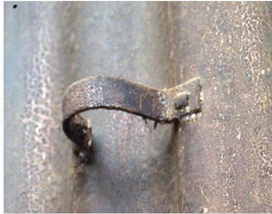
306 Bank Street, South Melbourne, gutter and downpipe brackets, believed to be original: Miles Lewis.
