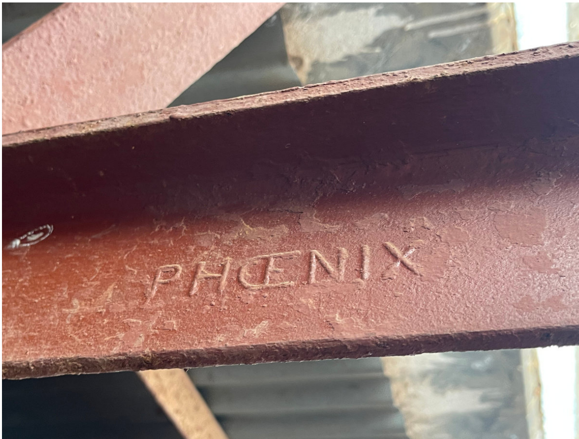
Phoenix rolling mark on a steel rafter: Tony Isaacson
