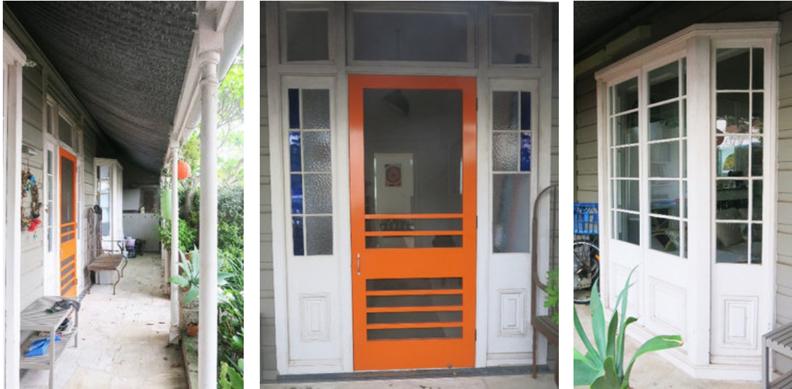
Verandah, with reconstructed roof and replicated columns: Miles Lewis.
