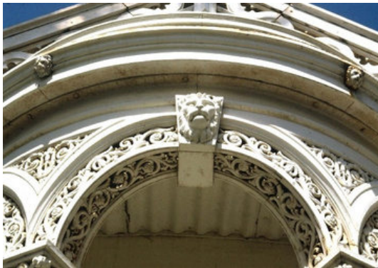
Corio Villa, details of the cast ironwork: Miles Lewis.
