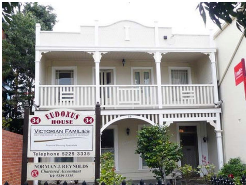
'Eudoxus', 34 Fenwick Street, Geelong, originally a semi-detached pair by John Walker, erected 1854: photo from the Victorian Heritage Register [cropped].
