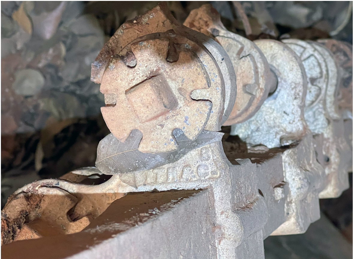
Cable equipment found below the floor: Tony Isaacson.
