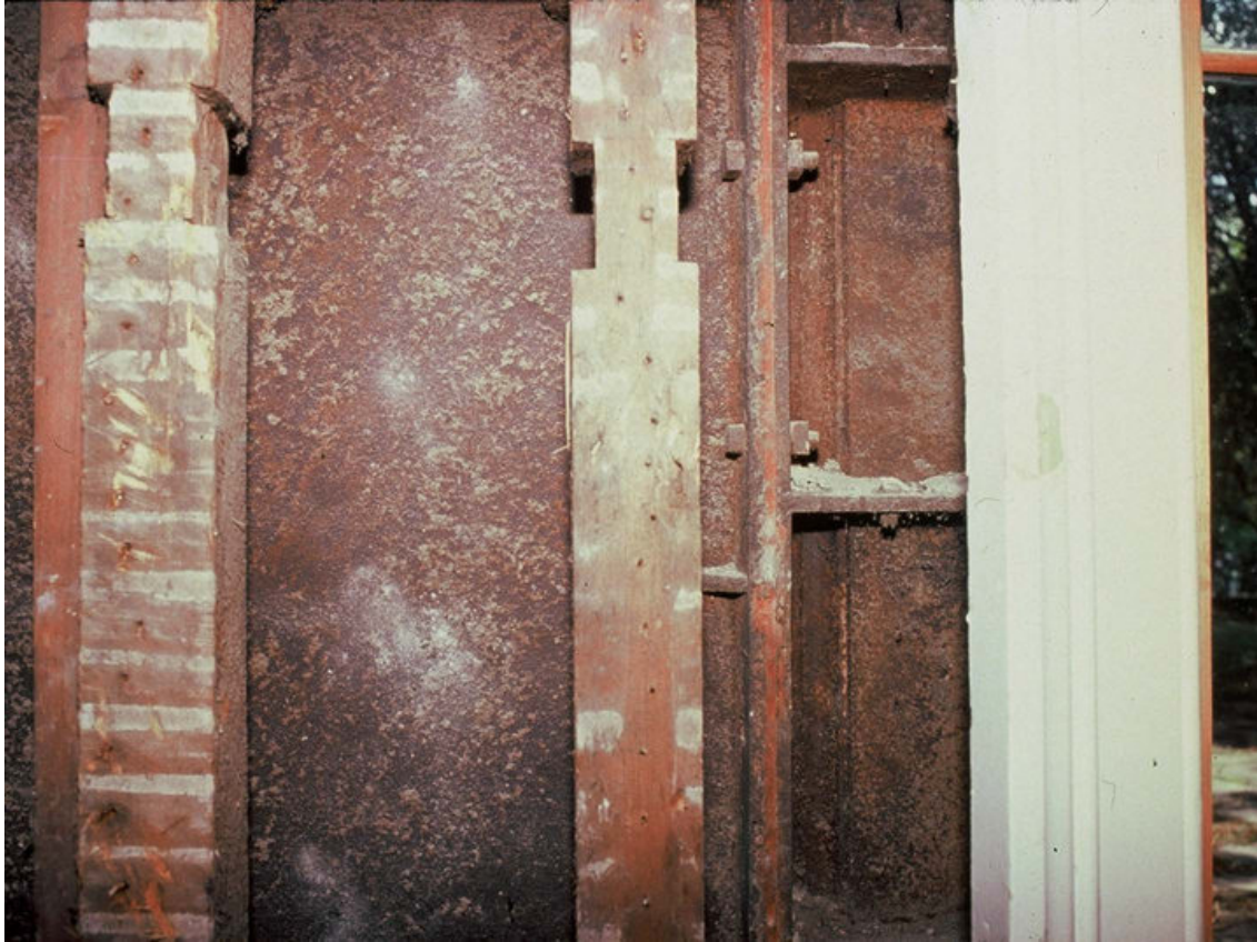
Corio Villa, Eastern Beach, Geelong, detail of the inside face of the west wall, showing timber studs stripped of lath and plaster, and behind these bolted iron tray construction. Miles Lewis.
