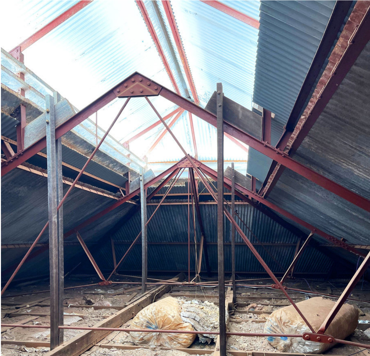
Roof space: Tony Isaacson.
