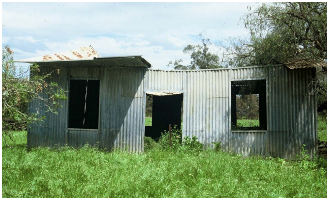
Iron house at 'The Weatherboard', Inverleigh, fabricated by John Walker, c 1853-4: Miles Lewis.
