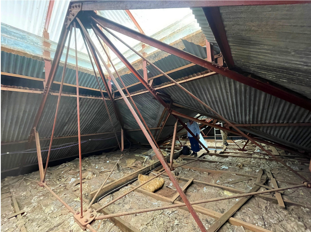
Junction of the main roof and the west roof: Tony Isaacson.
