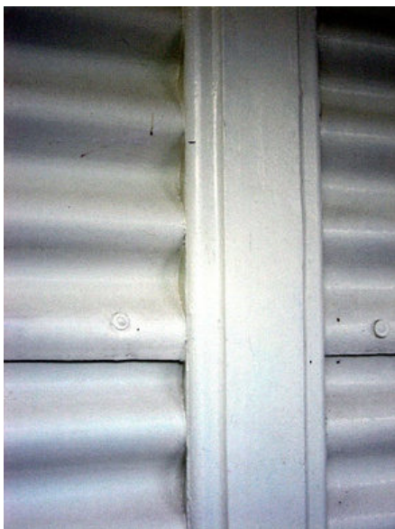
Corio Villa, detail of the corrugated iron rear wall, and diagram of the construction: Miles Lewis.
