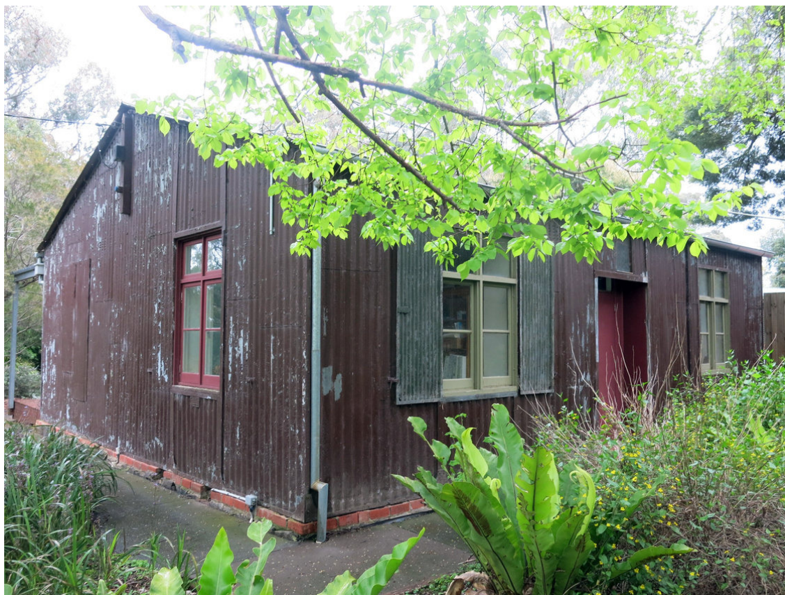
The ranger's house, 161-168 Gatehouse St, Parkville by [Benjamin] Walmsley (or John Walker) fabricated c 1853, erected by 1862: Miles Lewis.
