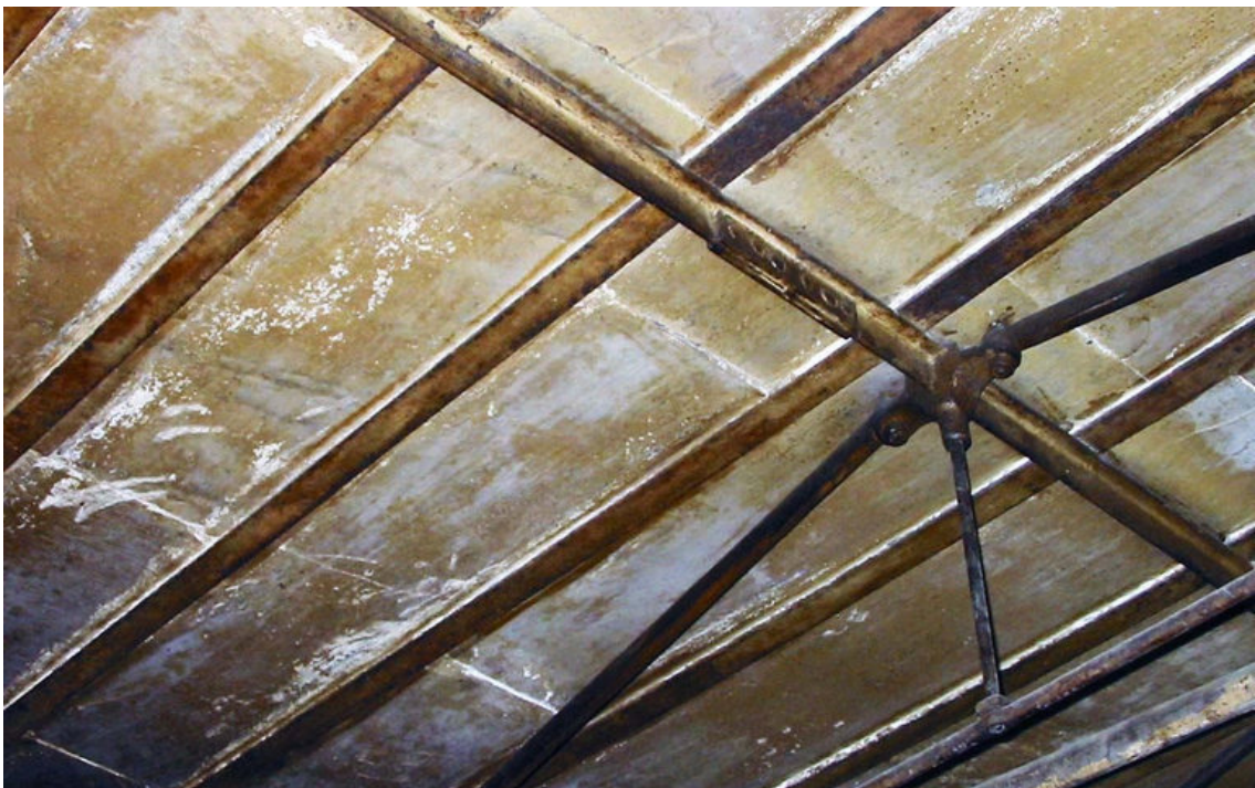
Royal Mint, Sydney, slate slab roofing: Miles Lewis.
