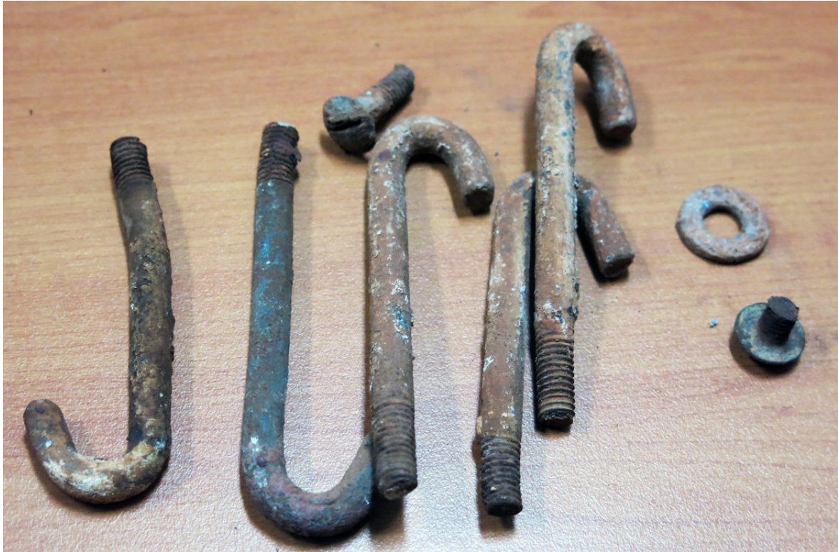
Hook bolts from the roof: Miles Lewis
