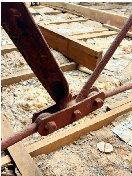
Truss bottom chord panel point: Tony Isaacson.
