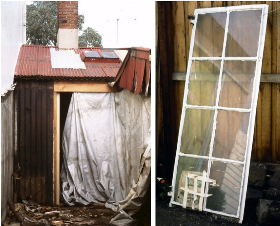
House at 306 Bank Street, South Melbourne, exposed rear wall as in 1983, and cast iron window sash: Miles Lewis.
