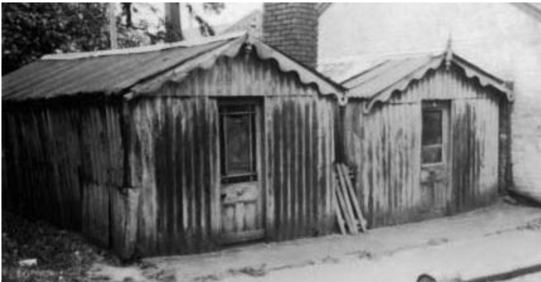
Two Hemming no 1 houses then surviving at 19 Byron St, North Melbourne, photographed by Oswald Barnett in the 1930s [detail]. Melbourne Library Service ID 18921.
