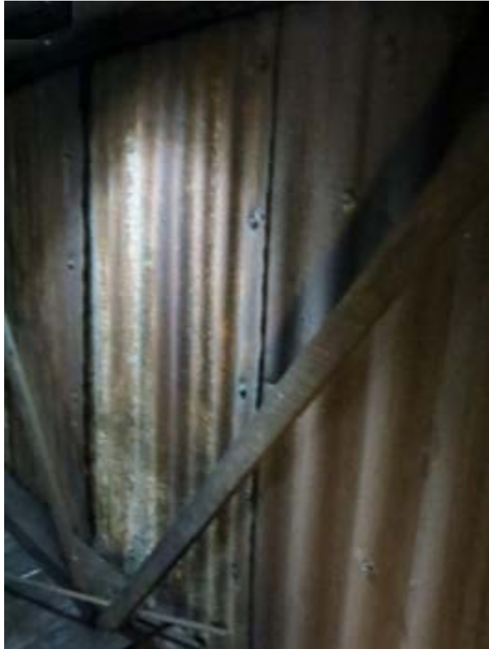
235 Rowntree Street, Birchgrove, stencilled timber formerly visible at entrance door sidelight: Jisuk Han. West gable cladding from inside the roof space: Miles Lewis.
