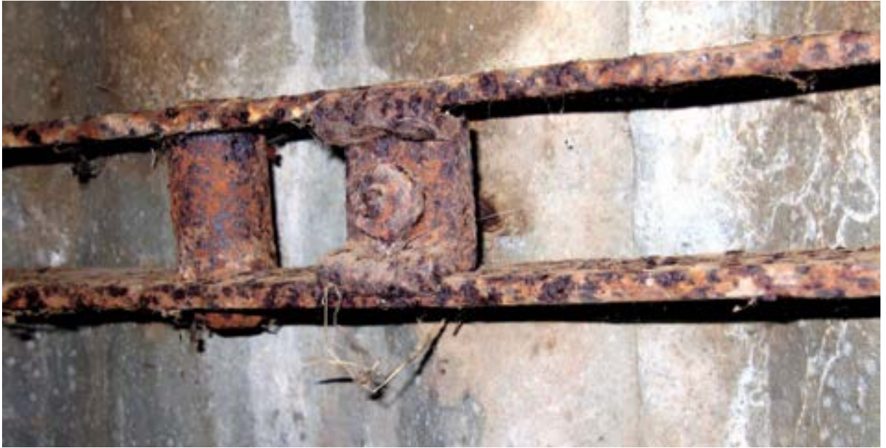
Iron building, Longford House, Longford, Tasmania, girt: Miles Lewis.
