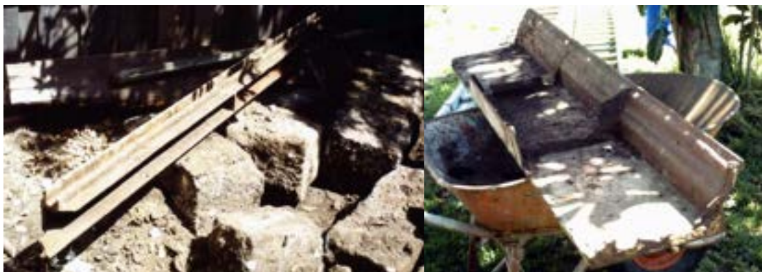
Corio Villa, a cast iron stanchion from the rear [corrugated iron] wall, and a cast iron gutter removed from the structure: Miles Lewis.
