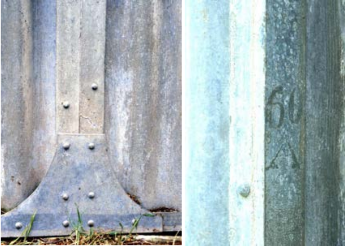
Details of the house at Inverleigh, gusset base joint, corner angle labelled '60/A': Miles Lewis.
