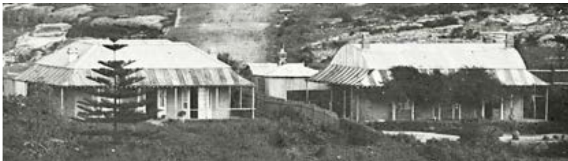
Two houses in Ballast Point Rd, Birchgrove, Sydney, with a hipped roof and a arched roof respectively, detail from the Panorama of Sydney from the Holtermann Residence c 1871-5, State Library of New South Wales ON Box 61 No C.
