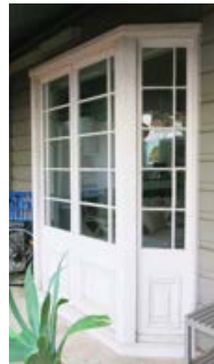
Verandah, with reconstructed roof and replicated columns: Miles Lewis. Front doorway, with largely original joinery: Miles Lewis. West window bay, central part reconstructed: Miles Lewis.
