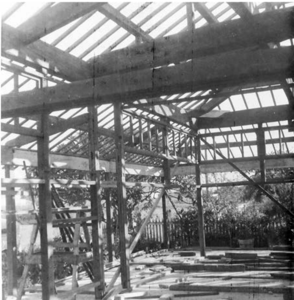
View of the house frame during dismantling: Markwell collection.
