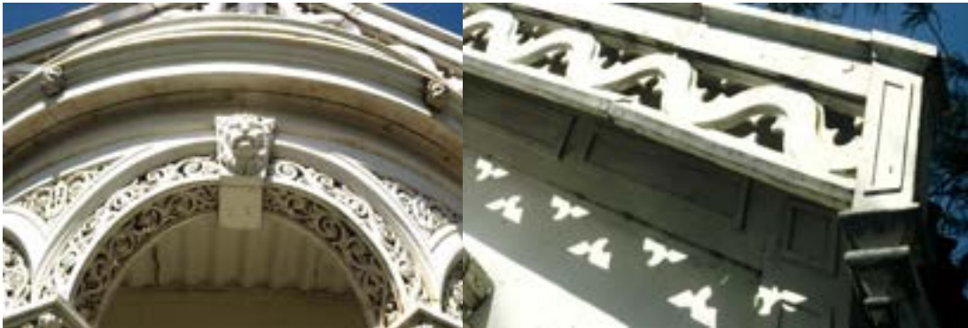
Corio Villa, details of the cast ironwork: Miles Lewis.
