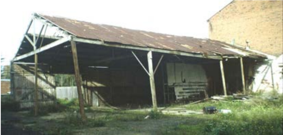
Store, rear of former Congregational Hall, 51 McKillop Street, Geelong, view prior to reconstruction. Photo, Miles Lewis.
