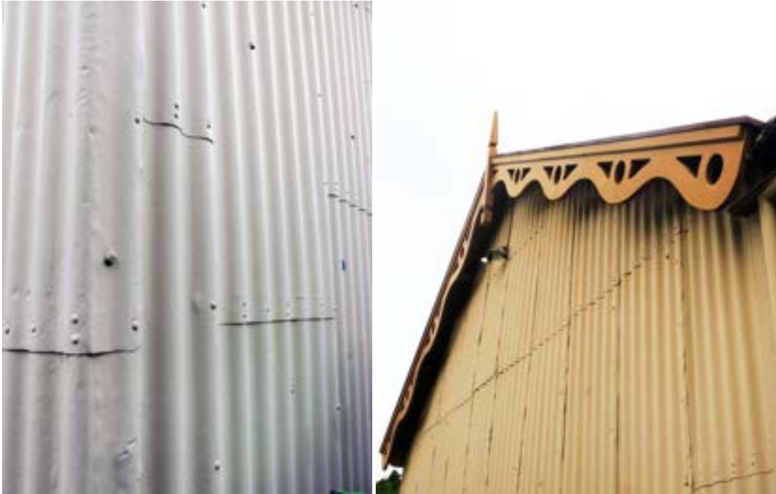
189 Brunswick Road, north wall cladding and gable: Miles Lewis.
