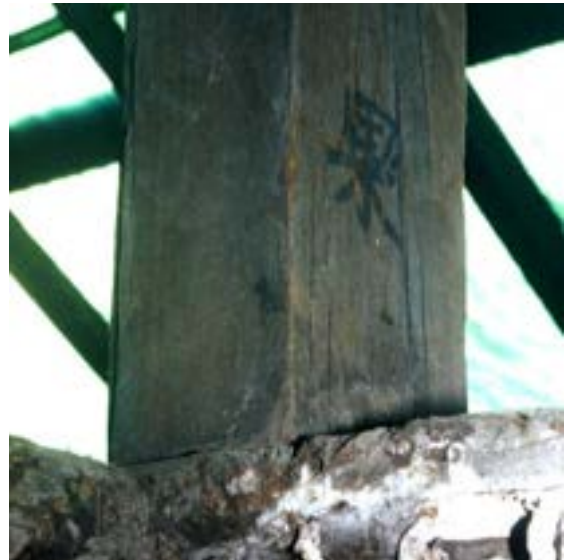
Details of the former 1 Hoddle St: (left) a hooked scarf joint in the base plate, over a stump (the left element decayed), (B) a roof strut or kingpost bearing a Chinese character: Miles Lewis.
