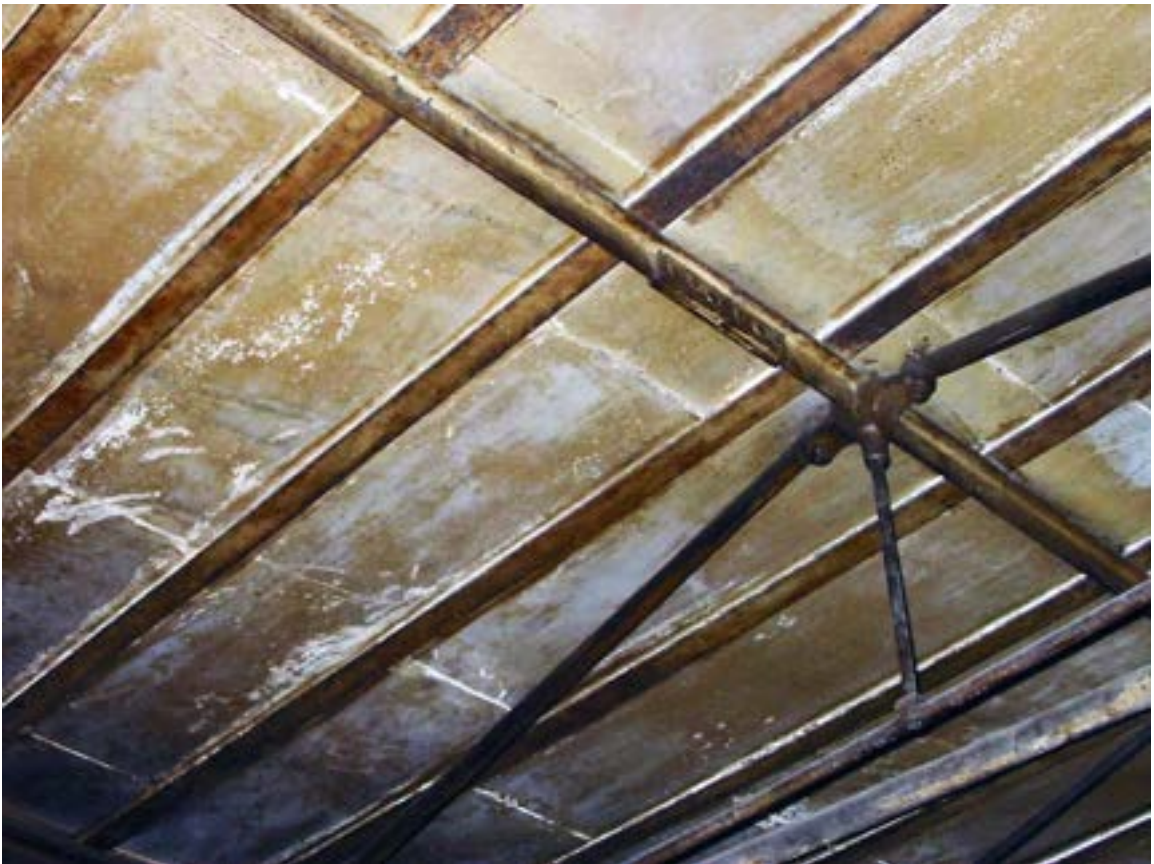
Royal Mint, Sydney, slate slab roofing: Miles Lewis.
