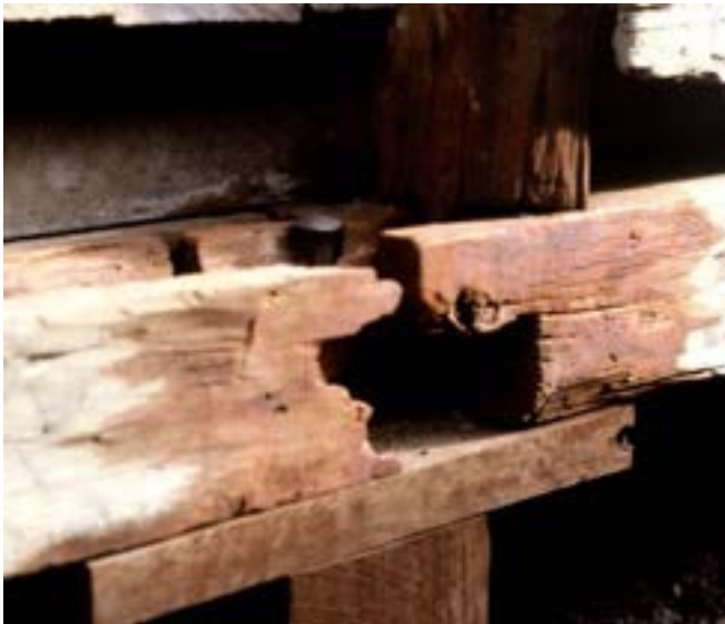
Details of the former 1 Hoddle St: (left) a hooked scarf joint in the base plate, over a stump (the left element decayed), (B) a roof strut or kingpost bearing a Chinese character: Miles Lewis.
