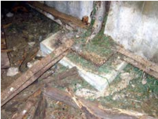
Iron building, Longford House, Longford, Tasmania, detail of the junction of a column base with a sub-floor tie and two base wall girts; lading mark on the corrugated iron: Miles Lewis.
