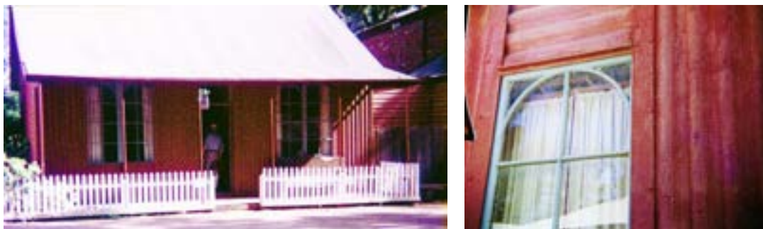
Iron house at the Swan Hill Pioneer Settlement, believed to be from the corner of Montague Street and Patterson Place: Miles Lewis.
