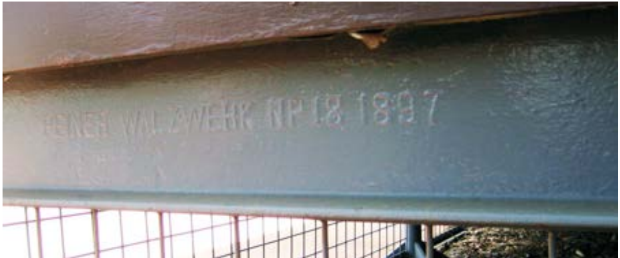
London and Hamburg Gold Recovery Company assay office, detail of the periphery beam showing the rolling mark: Miles Lewis
