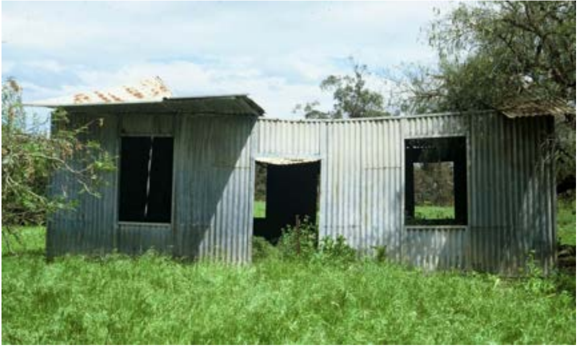
Iron house at 'The Weatherboard', Inverleigh, fabricated by John Walker, c 1853-4: Miles Lewis.
