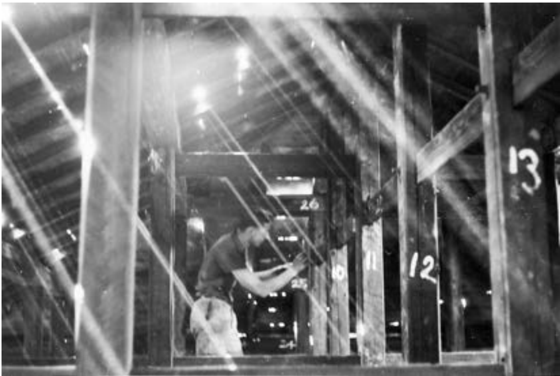
The roof framing: Markwell collection.
