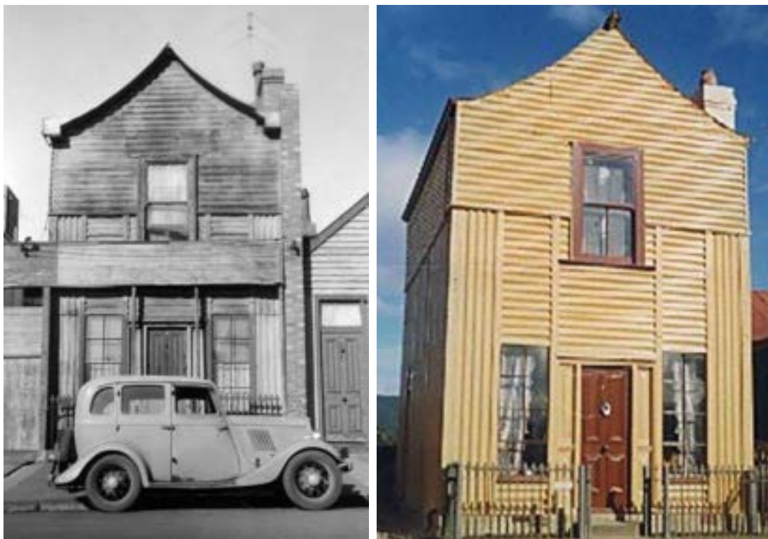
James Hogg house, formerly at 62 Curzon Street, North Melbourne, attributed to Robertson & Lister, c 1853, view on the original site in 1959: Clare Lewis & Mary Lloyd, 'Portable Buildings' (BArch, University of Melbourne 1959), plate 24B. As relocated at Old Gippstown, Moe: from the Old Gippstown web site, 2014.
