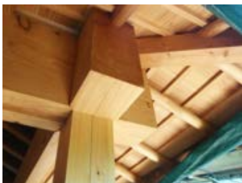
Details of restoration of the eaves and the gablet: Hugh Markwell.
