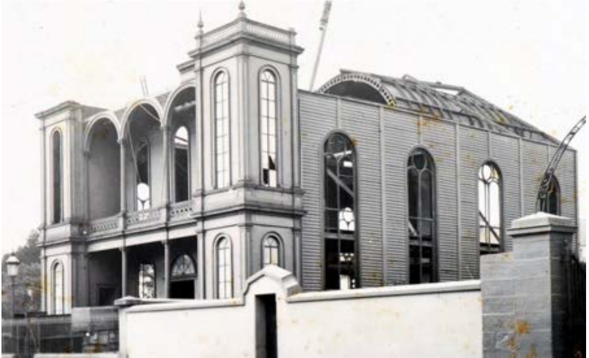
Former Free Presbyterian Church, Macquarie Street, Sydney, during dismantling, 1899: State Library of New South Wales PXE 1077 [cropped].
