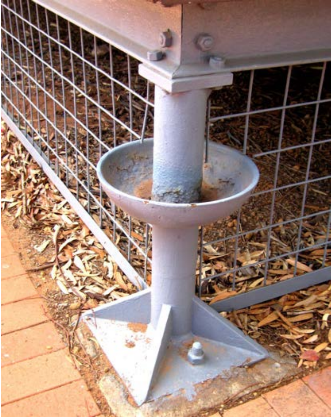
London and Hamburg Gold Recovery Company assay office, vermin-proof pillar: Miles Lewis
