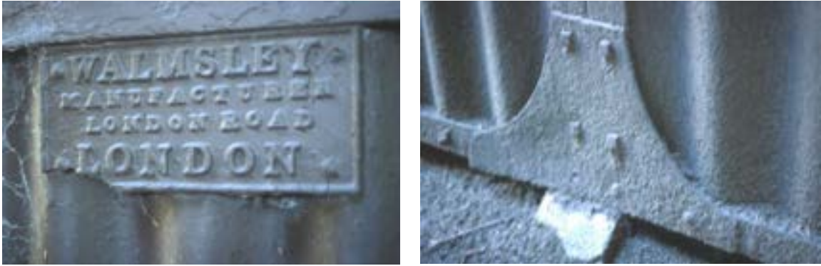
The ranger's house, Parkville, detail of the Walmsley plaque and a gusset connection: Miles Lewis.
