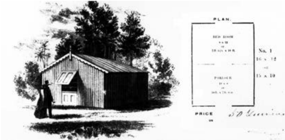
Cottage No 1 containing a bedroom and parlour, view and plan [reformatted]: Hemming's Patent Improved Portable Houses, Clift House, Bedminster: broadsheets held at the Baillieu Library, University of Melbourne.
