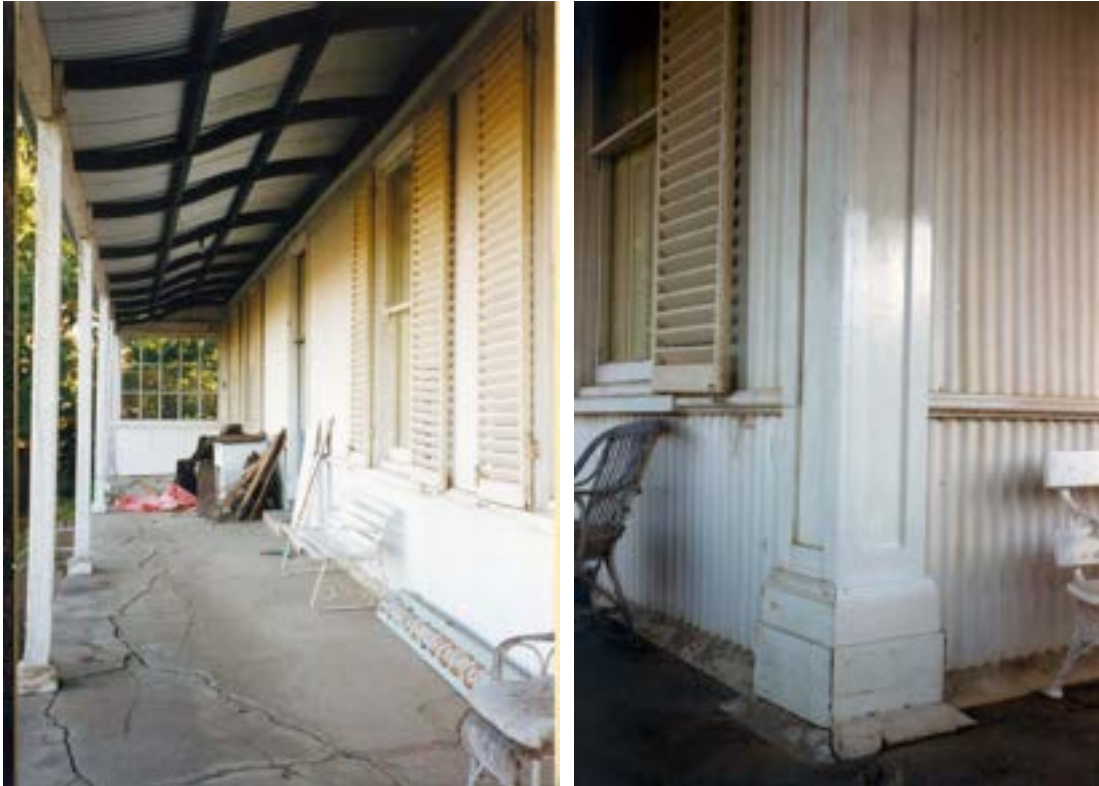
Wingecarribee verandah view: Miles Lewis. Corner detail: Bob Irving
