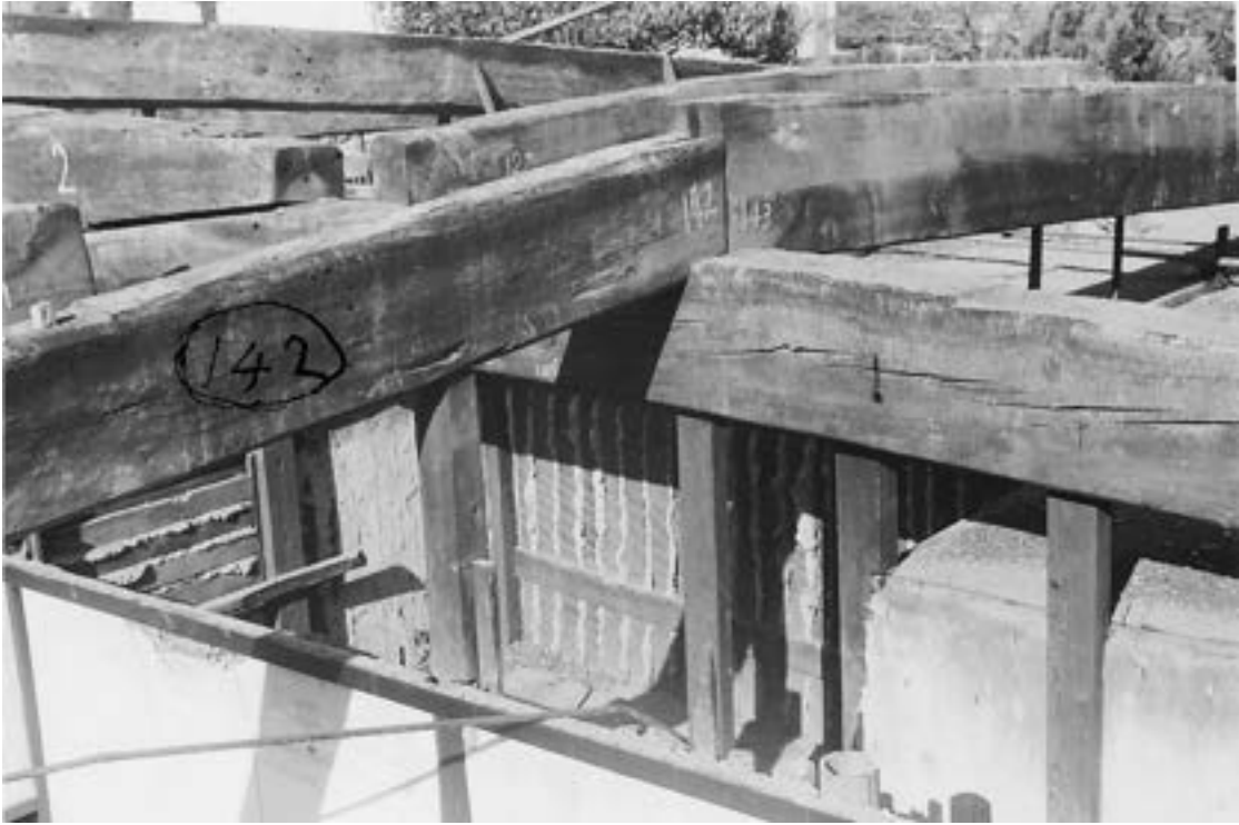
Detail of the roof structure during dismantling in 1962: Markwell collection.
