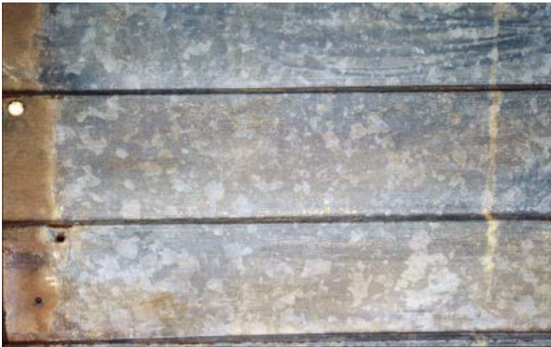
Wesleyan Church, Knuckey Street, Darwin, 1897: detail of imitation weatherboard cladding, seen from inside. Miles Lewis
