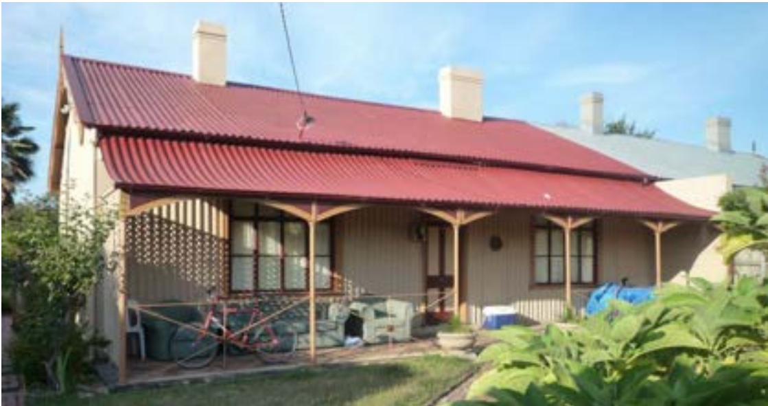
The most intact of the four houses. 189 Brunswick Road, Brunswick [Melbourne], 1854, attributed to Samuel Hemming.
