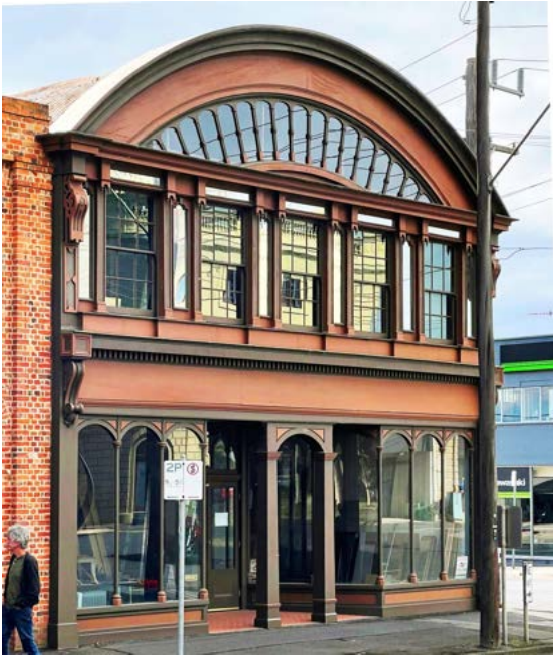
Brown Brothers store, front view as restored: Tony Isaacson.
