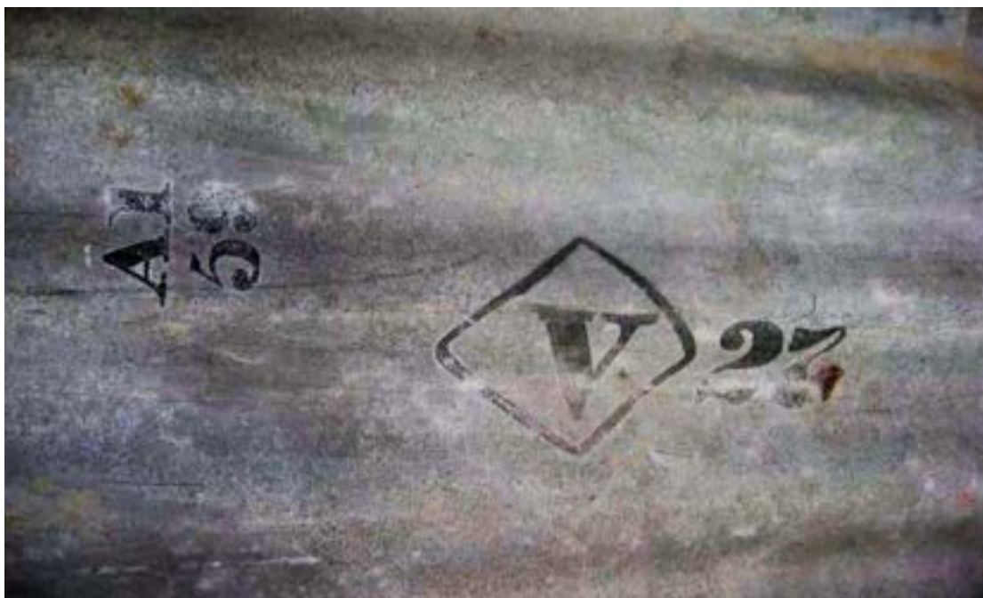
Marking on the iron of the Whanregarwen building, believed to be from the Melbourne General Post Office 1853: Natica Schmeder.
