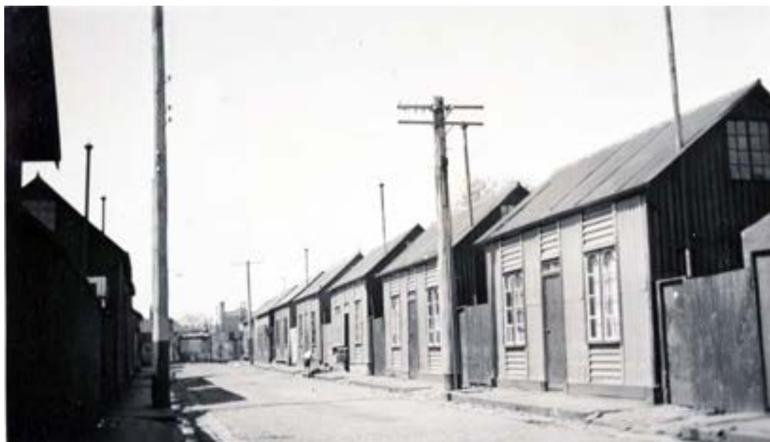
Patterson Place, South Melbourne, looking east, and showing the row of six iron cottages (nos 5 to 15) on the south side, 1933, photo by J K Moir. State Library of Victoria, no 819570.
